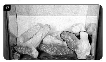
6.8 Sparingly spread an amount of the Embaglow fibres provided, covering the ports in the burner tray. Use a small piece in front of the log on the left hand side and a long strip in front of log B, see Diagram 18.
