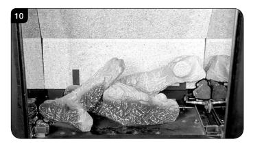
8.6 Log C rests on the cutout on Log E and is pushed up to the side and rear of the firebox, see Diagram 11.
