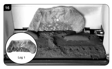
7.12 Place the second log into the left hand groove on the burner tray, see Diagram 17. The log should butt up against the raised molding and the left hand side liner.
