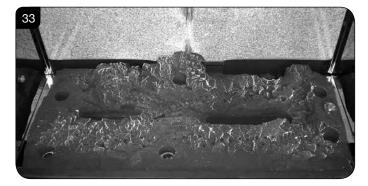
9.18 There are 3 embers. Place 2 embers in the back corners of the burner, resting in the cut outs, see Diagram 34.Place the last ember loosely at the front of the fuel bed to cover the hole in the centre.
