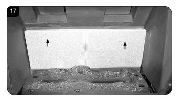
4.28 With the liners and baffle removed the firebox is clear for cleaning and maintenance, see Diagram 18.
