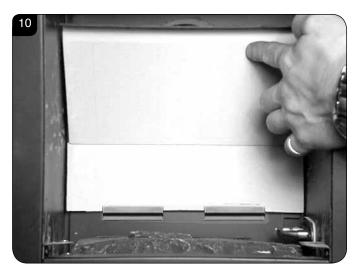
4.11 The lower rear liner does not need to be removed from the bracket in order to access the burner tray for maintenance, but can be lifted off in order to clean or replace, see Diagram 11.
