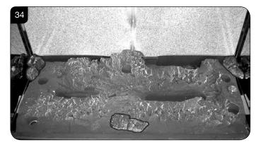
9.19 Place Log D on the left hand side of the burner. There is a hole on the underside of Log D which fits over the raised stud on the left of the burner. The back of the log should rest flat against the back panel, see Diagram 35.
